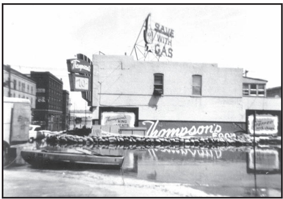
Frank and Mary Thompson started the Thompson Food Market in 1916. Advertising Thompson's as the "King in Meats," this 1965 photo shows the receding waters from the April flood which crested at an all-time high of 26.8 ft. The building in the far left background was the Tobert Drug Co (now Lot 1) and the other building, which now has a mural painted on the wall was the Schmidt Apartments (now 1st & Main). (Photo courtesy of the Loras College, Center for Dubuque History).
