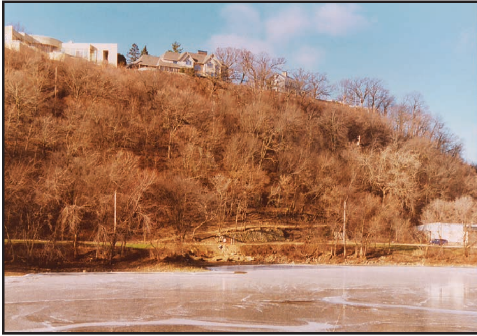
Today the smokestack is gone, but a paved Mt. Carmel Road winds down the side of the bluff near the location of the old smoke stack. (Photo by Terry Grant).
